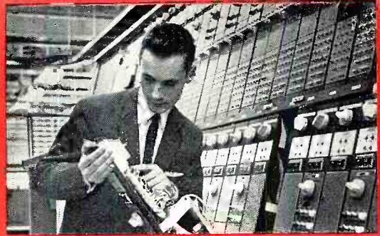
Checking panel wiring of Simplex console
